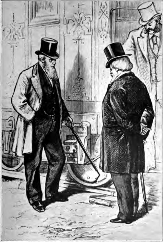
George M. Pullman explaining details of car construction
